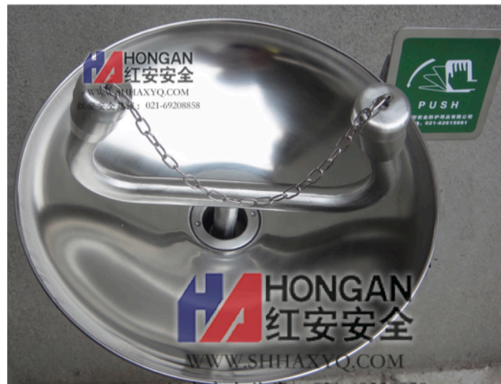
Figure 2. Eyewash with protective covers.
